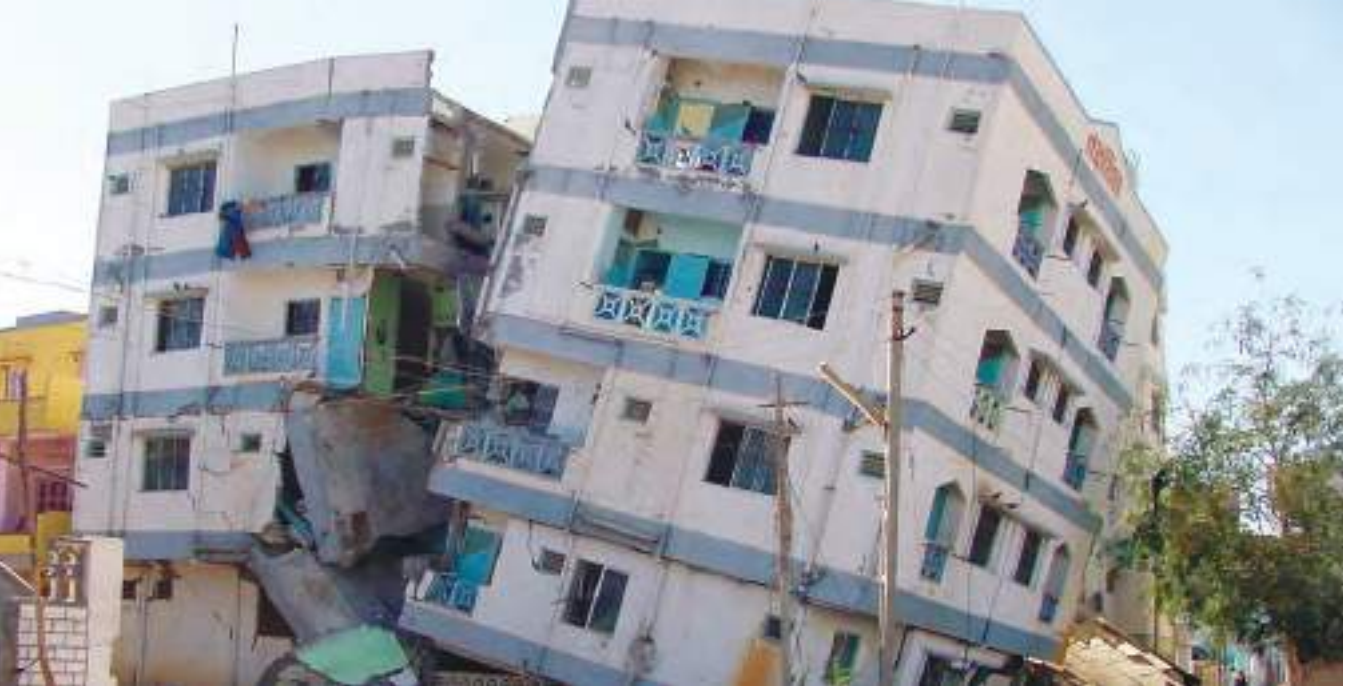
Damaged structure due to earthquake- Gujarat 2001
