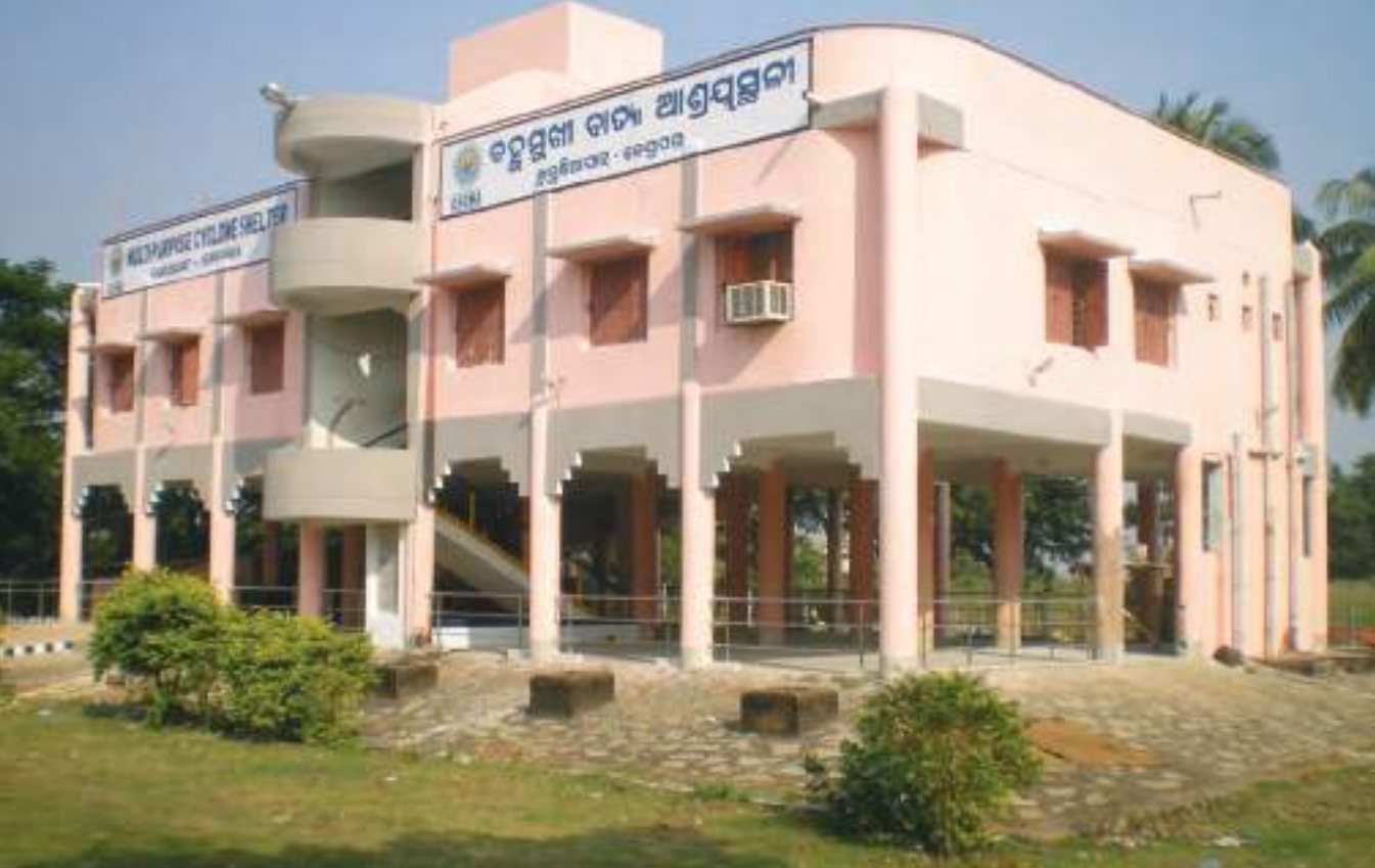
Multi-purpose Cyclone Shelter, Kendrapada, Orissa
