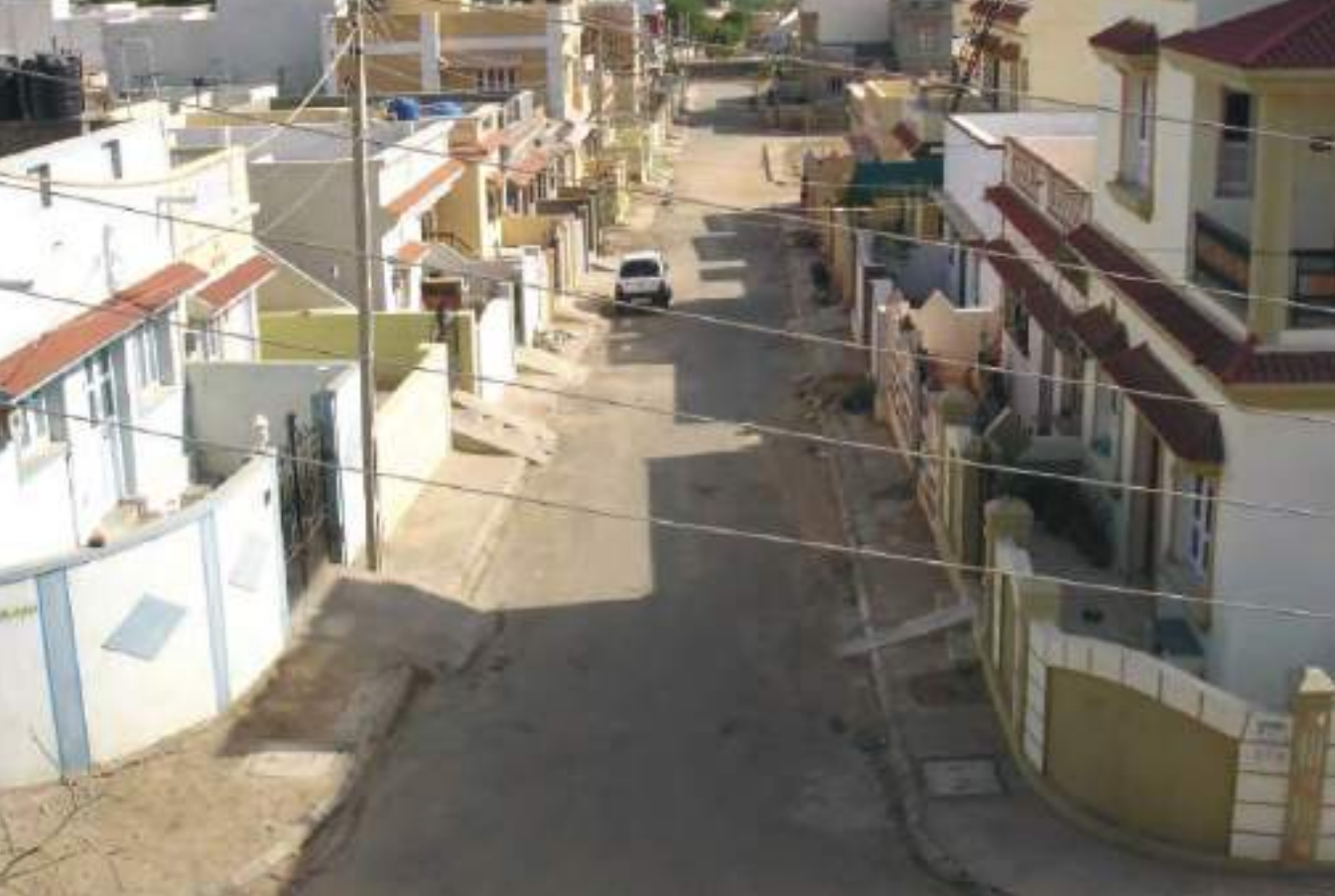
Kutch earthquake 2001 and reconstruction of house
