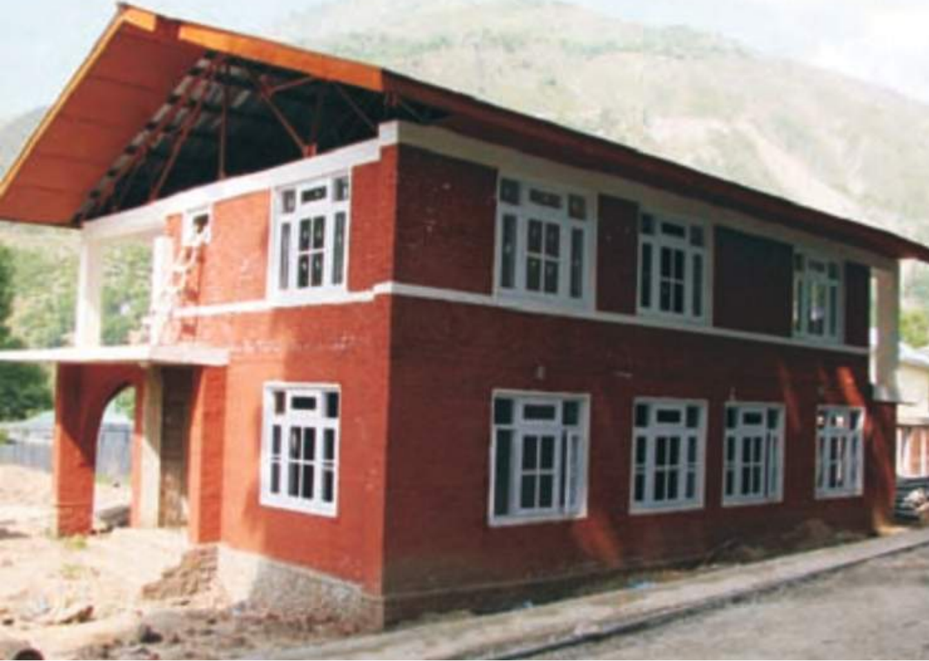
Jammu & Kashmir Earthquake 2005- Retrofitting on walls and windows
